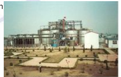
Laizhou Biogold Plant, China
