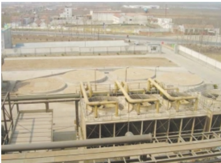
Biogold Bioleaching Facility, Laizhou, Shandong Province, China. View from the top of a Bactech bioleach plant. Note circular cement pads for future expansion (it is about to go to 150,000 oz/ly).
